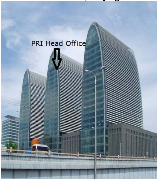
The PRI office building is located on top of 3 separate subways lines and Beijing North Railway Station, for convenient access all across the city
